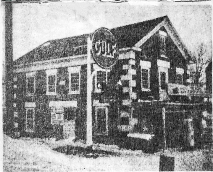
COBBLESTONE STORE AT PINE WOOD BUILT IN 1844
